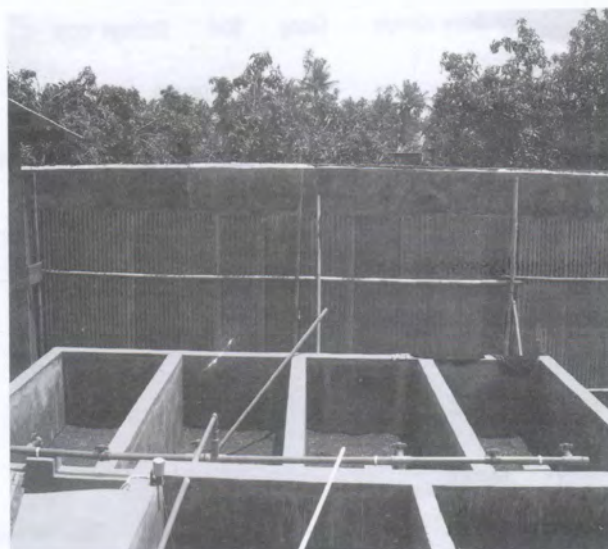
Gambar 4.29. Photo Unit Pengering Lumpur Secara Alami ( Sludge Drying Bed )
