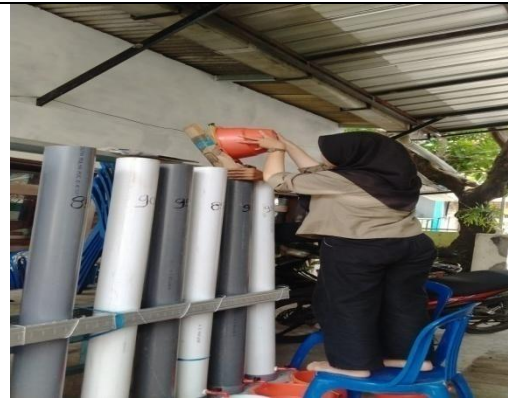
Gambar 10. Pengisian Media Kedalam Unit Adsorpsi
