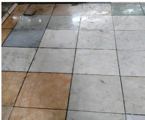
Lantai Ruang Proses
